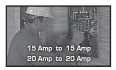
Make sure each circuit you move is protected by the same size breaker in the transfer switch. 15 Amp circuits must be connected to 15 Amp breakers and 20 Amp circuits to 20 Amp breakers.
